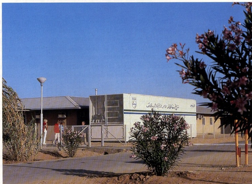
Fig. 1. PRX containerised exchange installed in Saudi Arabia
